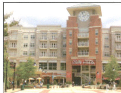
Pentagon Row in Arlington, Virginia, consists of 296,000 square feet of gross leasable area. It was built in 1999.
